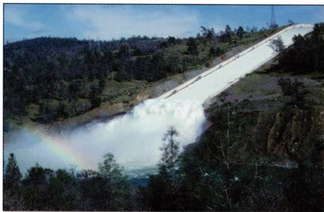
The Oroville Spillway helps maintain adequate flood control space.
