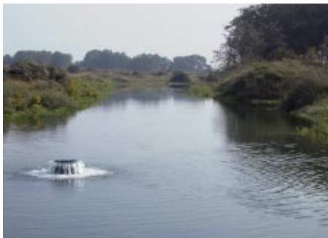
Saint André infiltration pond in Wulpen. © IWVA
